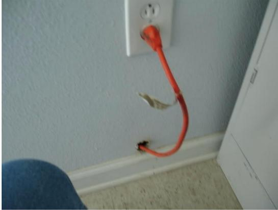
If you see something like this, which I have seen in homes that I inspect, find out where it goes and correct it. Either an outlet needs to be installed near the other end of this cord or some other correction needs to take place. Extension cords need to be completely visible from one end to the other.
