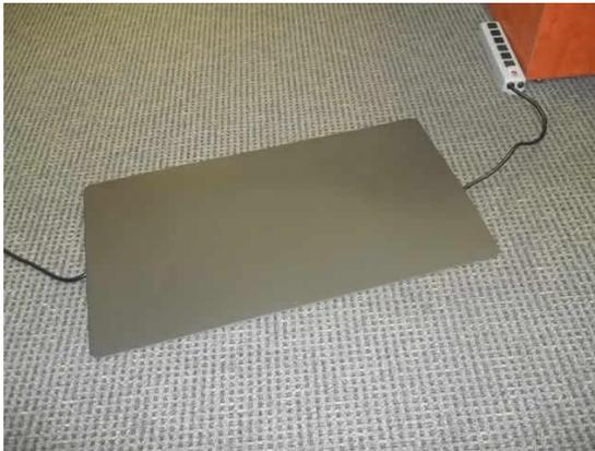
This is another hazard. I understand we want to make things safe and remove trip hazards but in doing this we increase the chances of the cord overheating and causing a fire hazard. Consider installing an outlet in the floor or relocating your electrical appliance.
